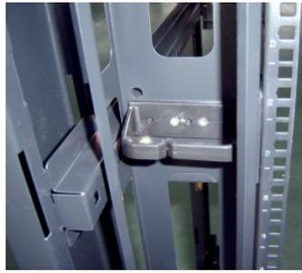
**2.7:** Installing the bayonet-type nut M6 on the spacer; and then using the allen screw M6x10 to connect the vertical cable management together tightly;
