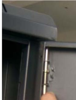
**2.7.1:** Installing the rotational pin for the back door on the bottom side; and then putting down bolt to aim the hole on the top, which is ok;
