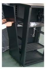
**2.8:** Chucking the clips to the middle of side panels by two hands, and then pushing the side panel to frame;
